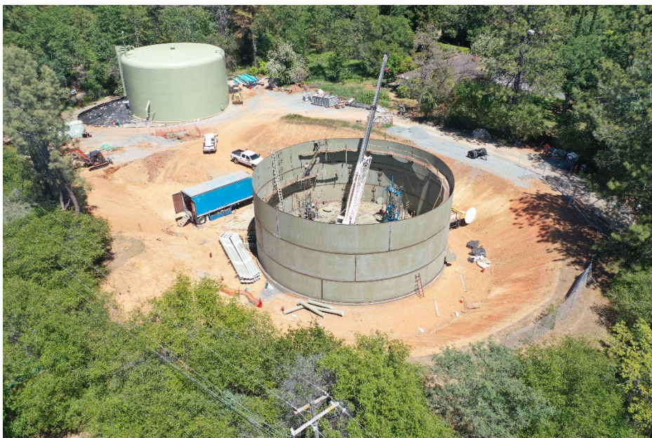
Tank 2 – Under construction looking to south towards Tank 1.
