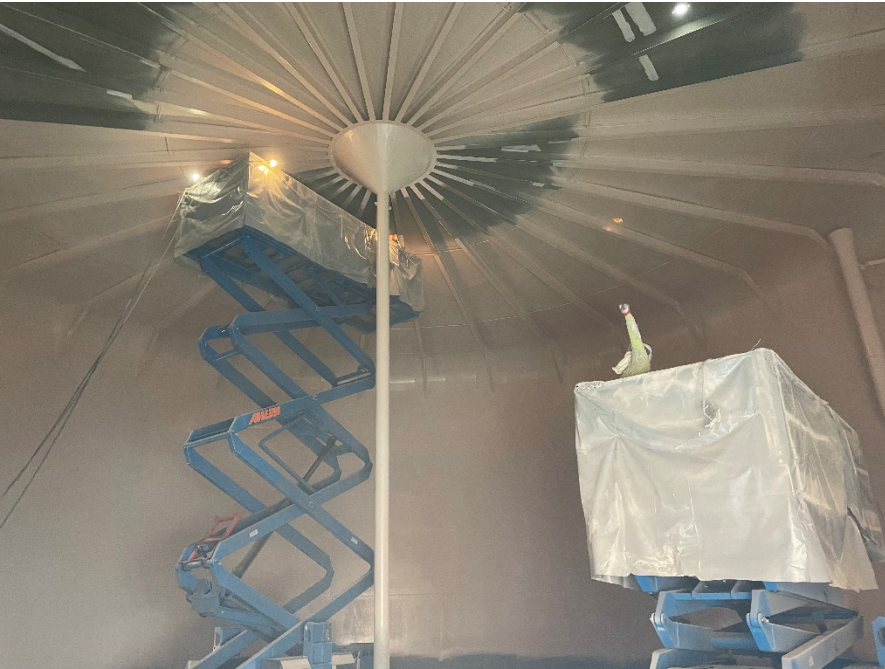
Intermediate coat - note pink tint to distinguish from top coat (white)
