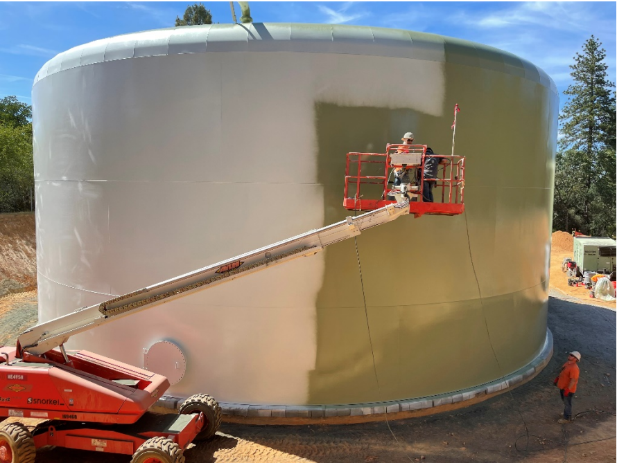
Exterior painting - top coat (green) over intermediate coat (white)
