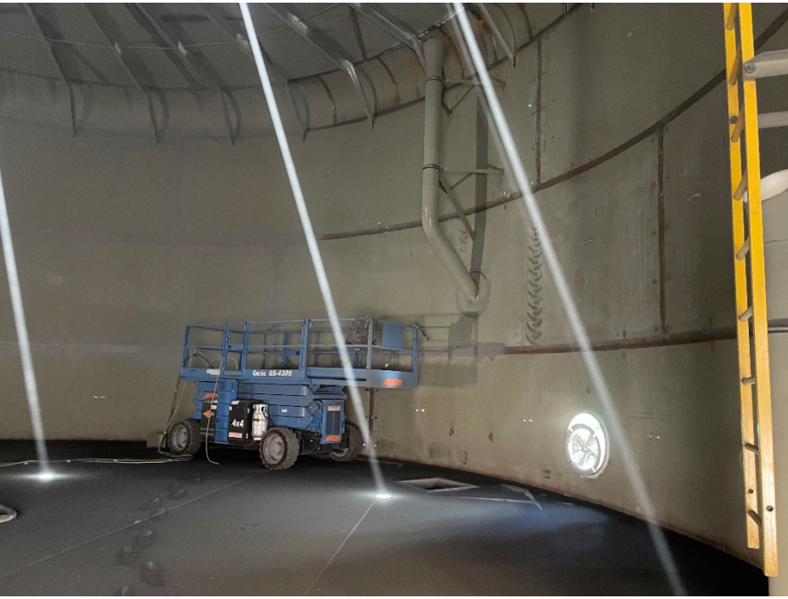
Interior of Tank 2 - Sand blasting and prepping for stripe coat
