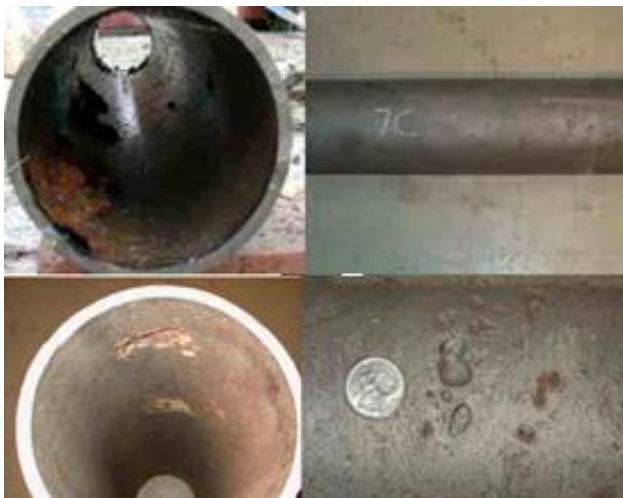
6" Cl pipe with 10% measured loss
