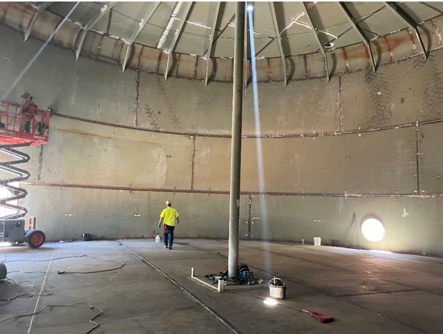
Interior of Tank 2 prior to coating – green color is the zinc primer
